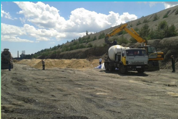
Recultivation works on the dump slopes
